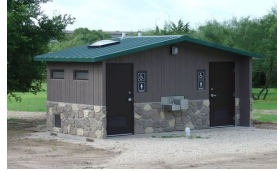
Fryer Park Restroom
