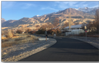
“GREAT” pavement conditions are marked by smooth, unobstructed pavement with none to minimal amount of distress.
