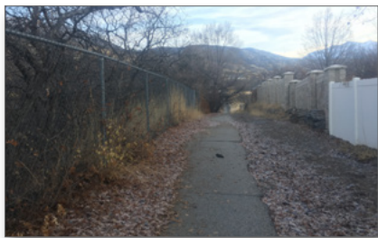
“POOR” pavement conditions are marked by rough pavement quality with significant obstructions, such as branches, leaves, and other debris, with moderate to significant amounts of distress.
