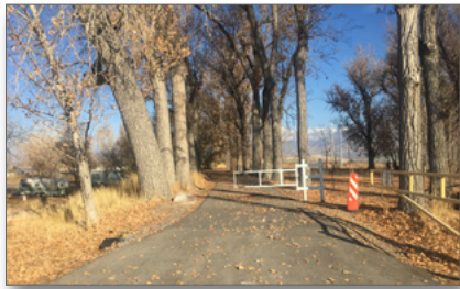
“GOOD” pavement conditions are marked by relatively smooth, unobstructed pavement with minimal to minor amounts of distress.
